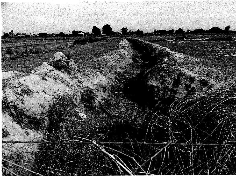
Picture of ditch through Juan Sanchez's property. Top width of ditch approximately 17 feet. Bottom width of ditch approximately 6 feet.
